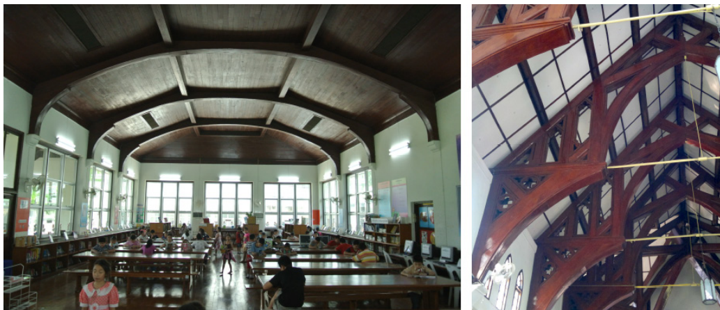
Figure 7. The inside of Power Hall (built in 1928), using the Wooden Rigid Frame Structure to maximize the width of the building. Today it functions as a library.
