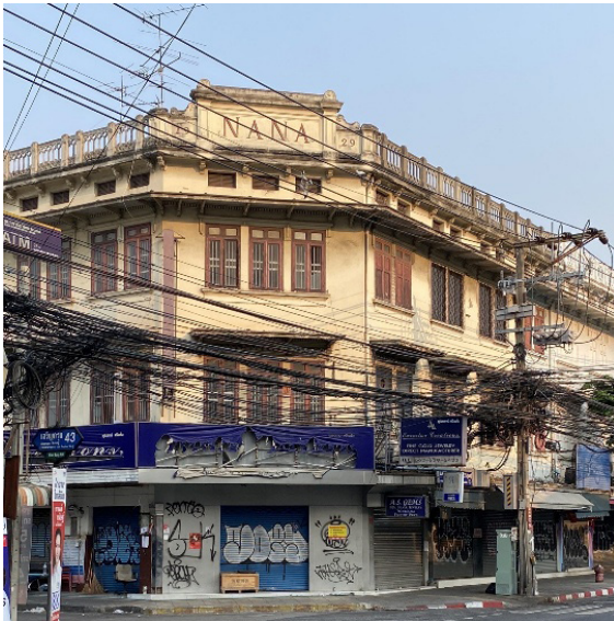
Figure 3. Cluster of old buildings Source: Author.
