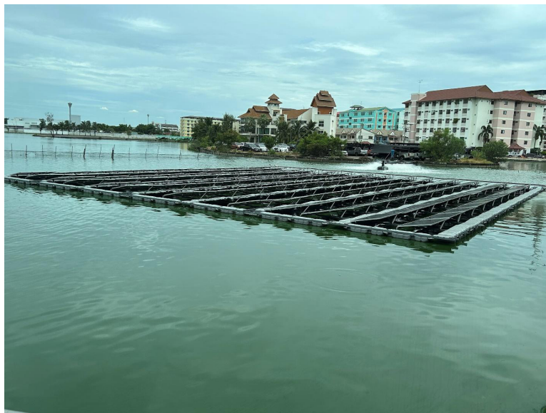
Figure 12. Recently-installed floating PV solar power system on the pond in the heart of Nava Nakorn (photo by authors).
