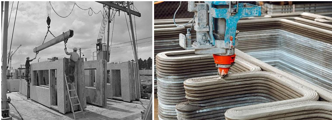
Figure 4. Economy of scale with pre-cast wall units minimizing construction cost (left). 3-D printed wall elements eliminating the need for formwork in new fabrication logic (right). (Source: left - -Sokołowski, (1970, as cited in Tsimer, 2018) / PAP; right - Vu and Iso (2022))
