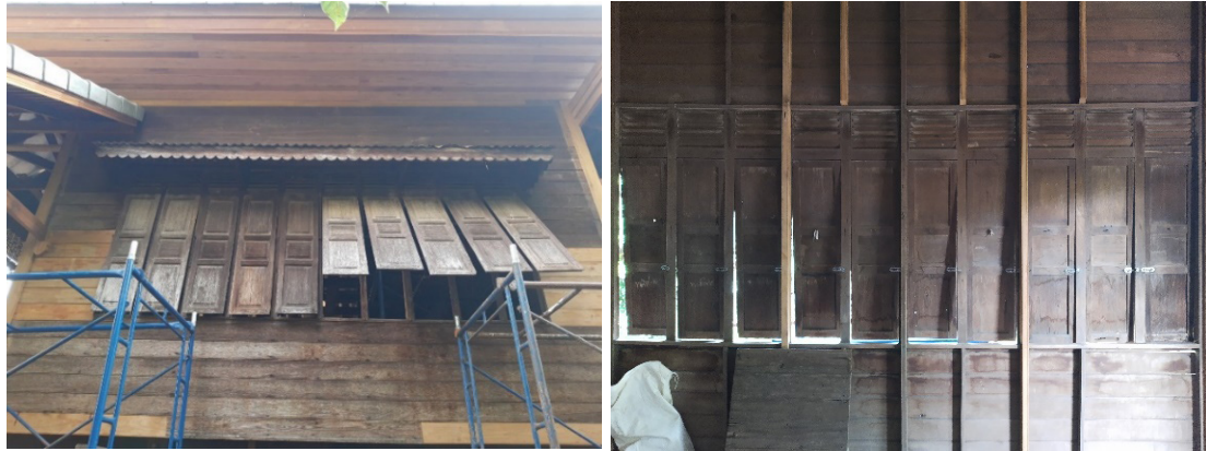
Figure 14 Replacing the damaged facade with new wood (Credit: North Forest Studio)
