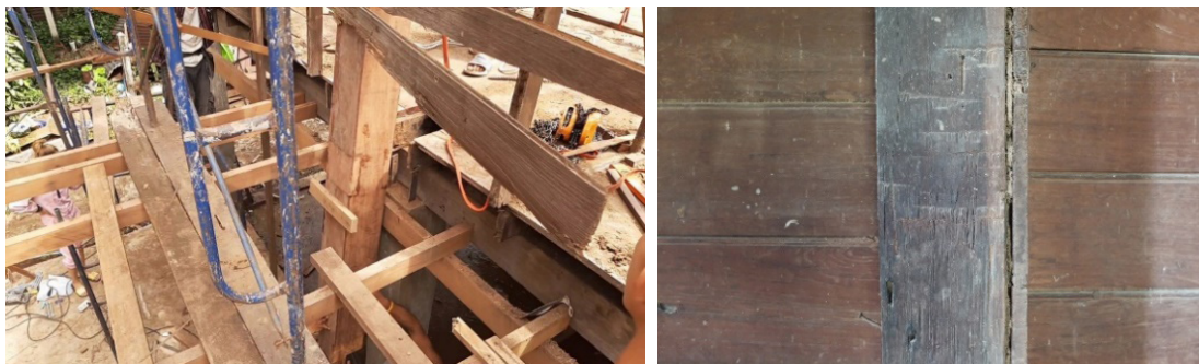
Figure 11 Different levels in interventions: changing columns and replacing wood in joists (Credit: researcher)
