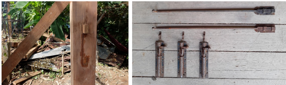
Figure 15 Inventive intervention of joints and the reusable accessories (Credit: (left) researcher, (right) North Forest Studio)
