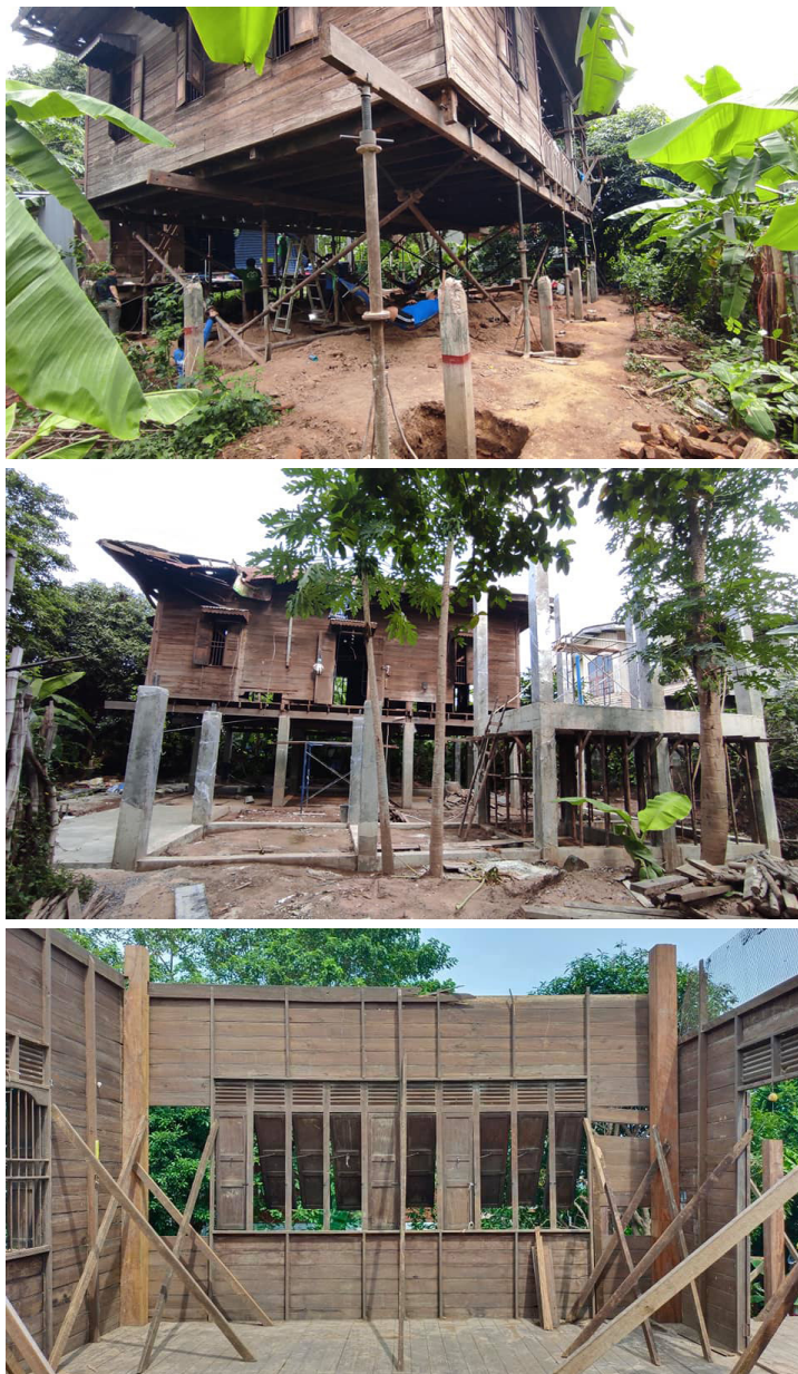
Figure 5 The three phases of the renovation process; (top) lifting the house, (middle) rebuilding the service zone, and (bottom) wood reconstruction and repair (Credit: researcher)
