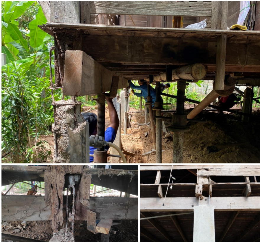
Figure 9 An unplanned situation resulting from the sign of a cracked beam during house lifting (Credit: researcher)
