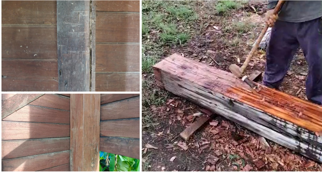
Figure 12 Old and new column texture and an adze (Credit: (left) researcher, (right) North Forest Studio)
