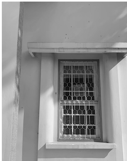
Figure 9 Wrought-iron Burglar Bars on the Front Windows.
