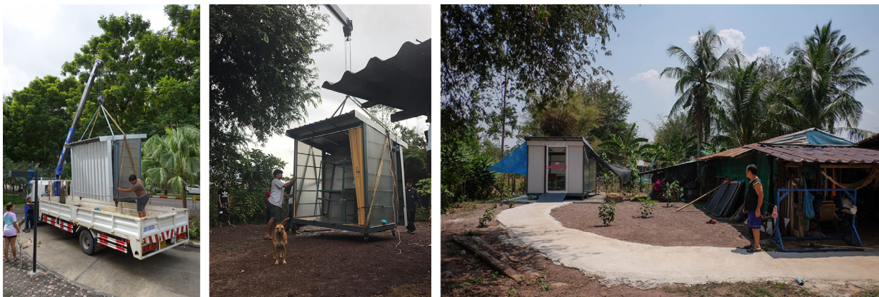
Figure 8. Unit delivery and installation on site
