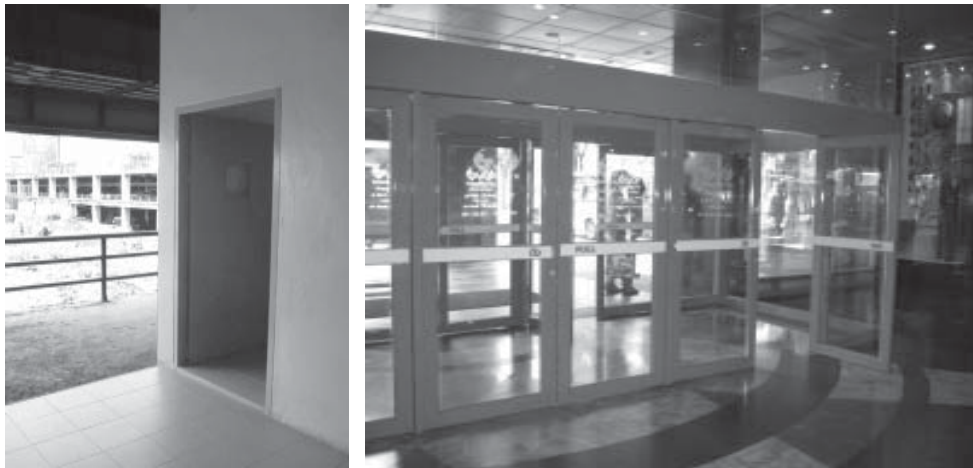
Figures 12 and 13 In some public buildings, little things like switching door swings in the direction of egress can easily save more lives during an evacuation. Design professionals should pay more attention to codes and to what makes sense.
