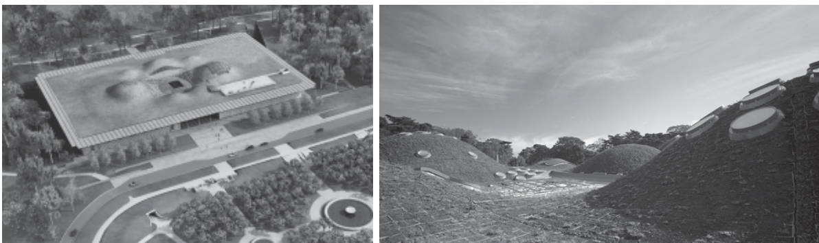
Figure 11. Extensive green roof of LEED platinum winner, California Academy of Sciences, designed by Renzo Piano.
