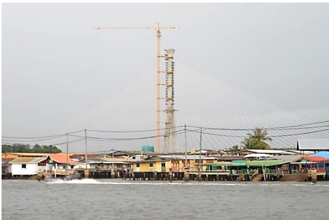
Figure 7 Bridge construction project to across Brunei river
