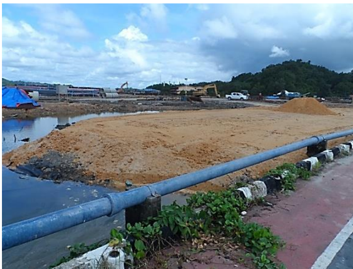
Figure 6 Filling soil to expand area after demolition Sungai Kedayan village
