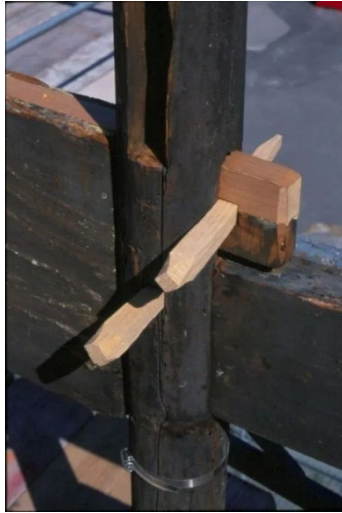
Figure 7: Mortise and tenon joinery at Yin Yu Tang (Story FM, 2023)
