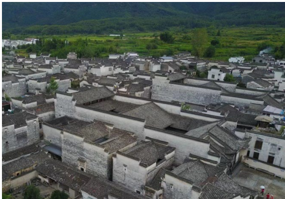
Figure 9: The roof of Huizhou architecture (Shot by Chen Juan in 2023)
