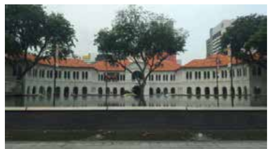
Figure 12 A building in Singapore
