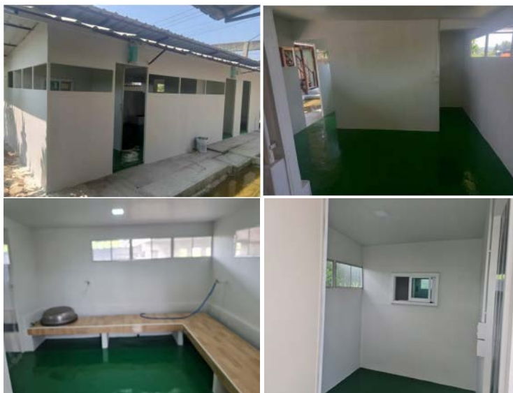
Figure 9. Raw material preparation rooms, raw material storage rooms, frying rooms, and packing rooms
