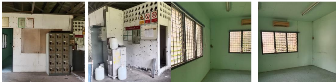
Figure 2. Pre-renovation of kombucha production area Source: Siam Phomprathan Co., Ltd.
