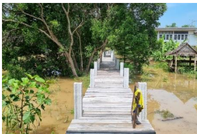
Bridge along the canal
