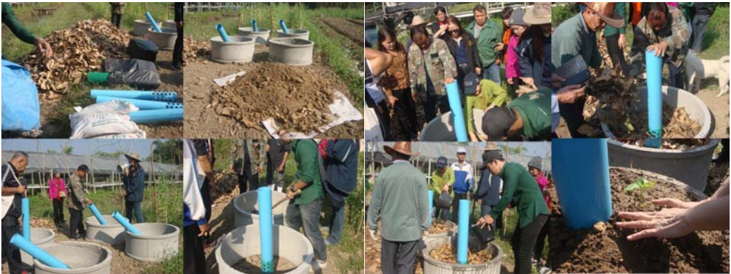
Figure 2. Keyhole garden construction under participatory with community
