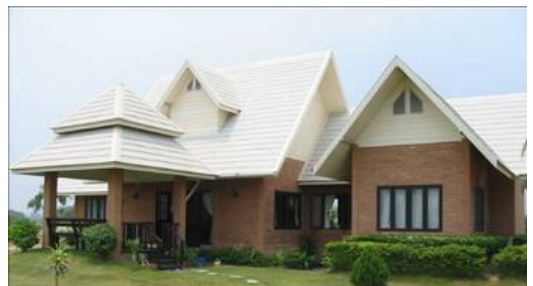
Figure 2 Interlocking block usage
